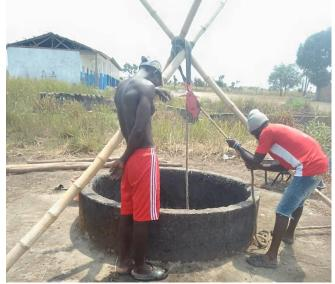
The next task was to form a concrete top for the well which includes an inspection cover to give them access for any future repairs and the also a pipe which houses the pump handle mechanism. The completion of the well took place on Sunday April 14<sup>th</sup>, meaning that the entire project took just 3 weeks, which is very impressive when you remember that everything is done manually.
